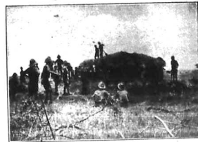
RHODESIANS BUILDING BLOCK HOUSES
