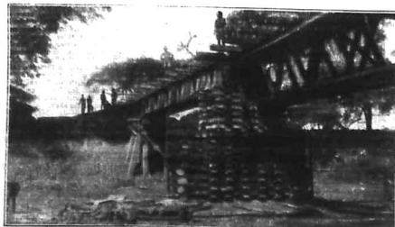
A TEMPORARY BRIDGE CONSTRUCTED IN RECORD TIME OVER THE WARA-WARA.
