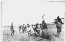
NATIVES LAYING DOWN "PIPE LINE" IN "GERMAN" EAST.
