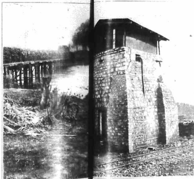
A GERMAN BRIDGE NEAR THE USAMBARA WATER TANK AT BURO STATION.
