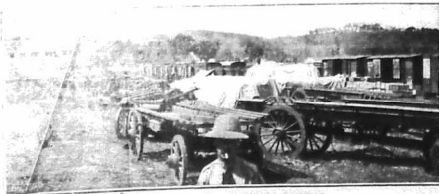
MAUZI STATION ON THE USAMBARA RAILWAY.
