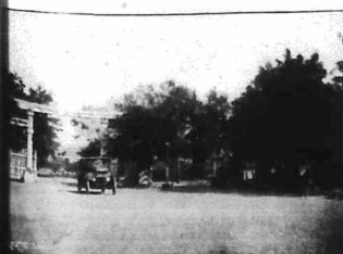
ENTRANCE TO MWANZA BARRACKS.
