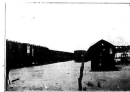
M'BUYUNI RAILWAY STATION. The station itself is made from an aeroplane parking shed. Photo: W. B. FRANK, Nairobi.
