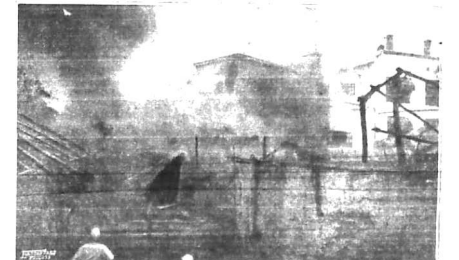
THE FIRE AT THE EAST AFRICA HOUSE, ON SUNDAY MORNING, JUNE 23RD, SOON TOO HAD ALARMING DIMENSIONS. THE POLICE WERE EARLY ON THE SCENE AND WERE SUCCESSFUL IN BRINGING THE FIRE EVENTUALLY GOT UNDER CONTROL. THE DAMAGE IS ESTIMATED AT WELL OVER £100,000.
