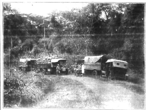
AFTER A COLLISION AT A BAD CORNER ON THE KAMPALA-TORO ROAD
