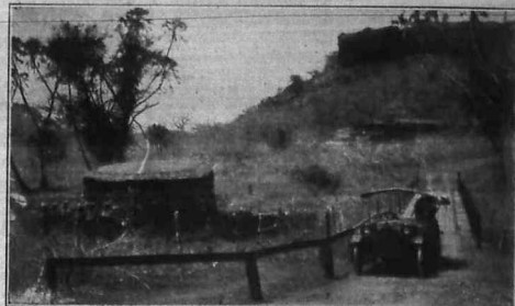
4 MILE BRIDGE, TSAVO-TRAMBO ROAD.
