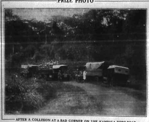
AFTER A COLLISION AT A BAD CORNER ON THE KAMPALA-TORO ROAD
