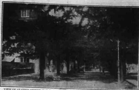
VIEW OF ARATTEN STREET, DAR-ES-SALAAM, SHOWING Y.M.C.A. BUILDING, ON THE LEFT.
