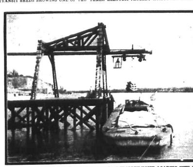
ONE OF THE THREE PIER HEADS SHOWING ELECTRIC-TROLLEY-HOIST LOADING INTO LIGHTER.
