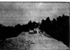
THE ROAD BEING MADE THROUGH A MANGROVE SWAMP.
