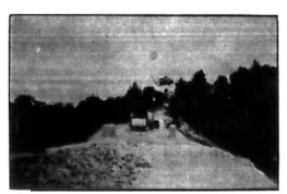
THE ROAD BEING MADE THROUGH A MANGROVE SWAMP.
