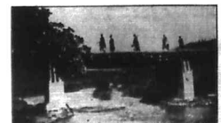
TAMBARA BRIDGE—MYRI IN USE
