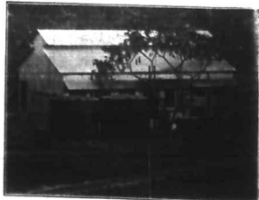
THE NEW ELECTRIC POWER STATION AT SHIMANI, MOMBASA, KENYA COLONY.
