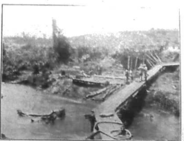
THE BRIDGE AT THAIKA
