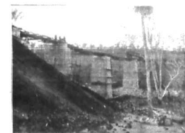
THE BRIDGE AT THAIKA
