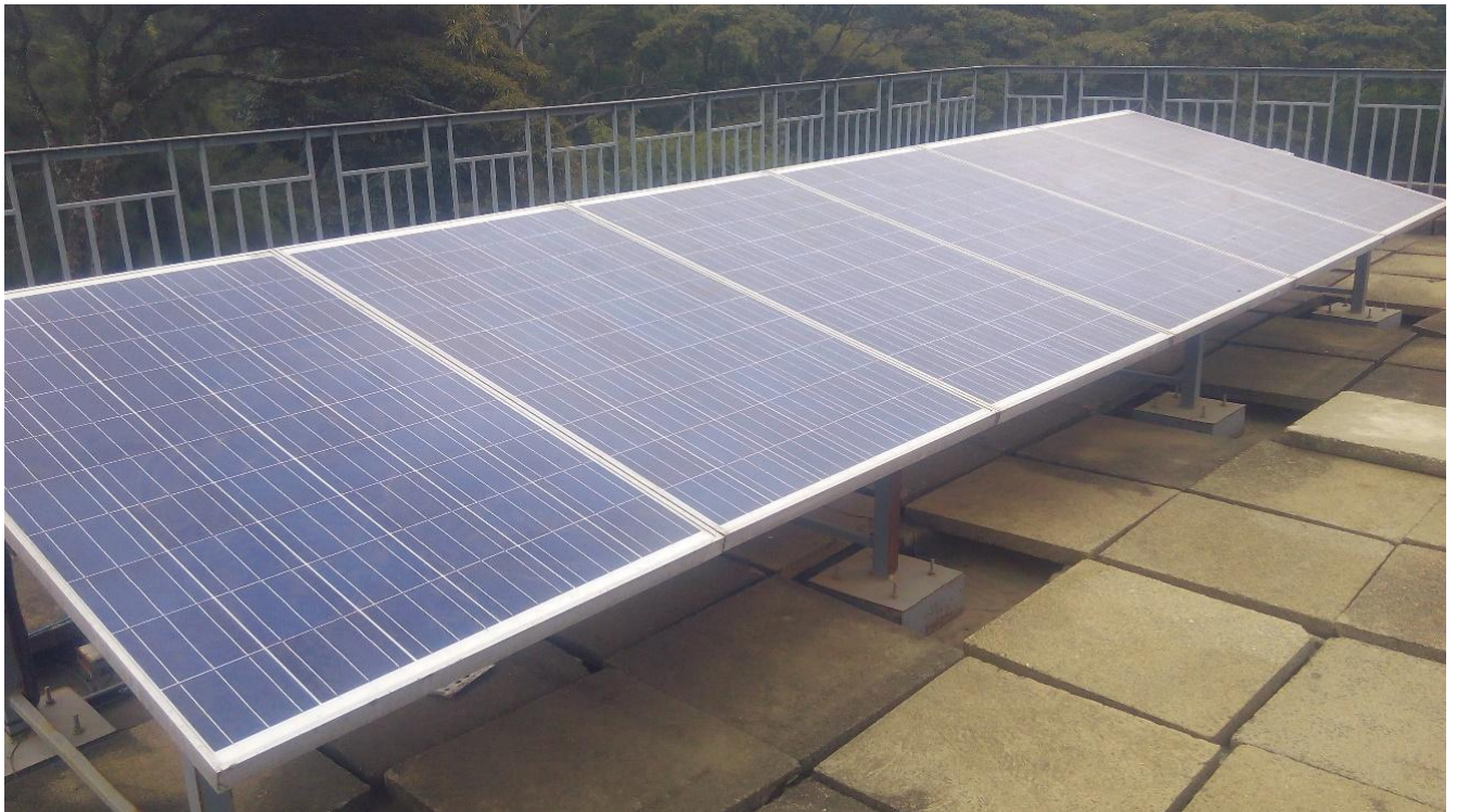
Figure 4.1: Image of the 1.5kW PV Module station
