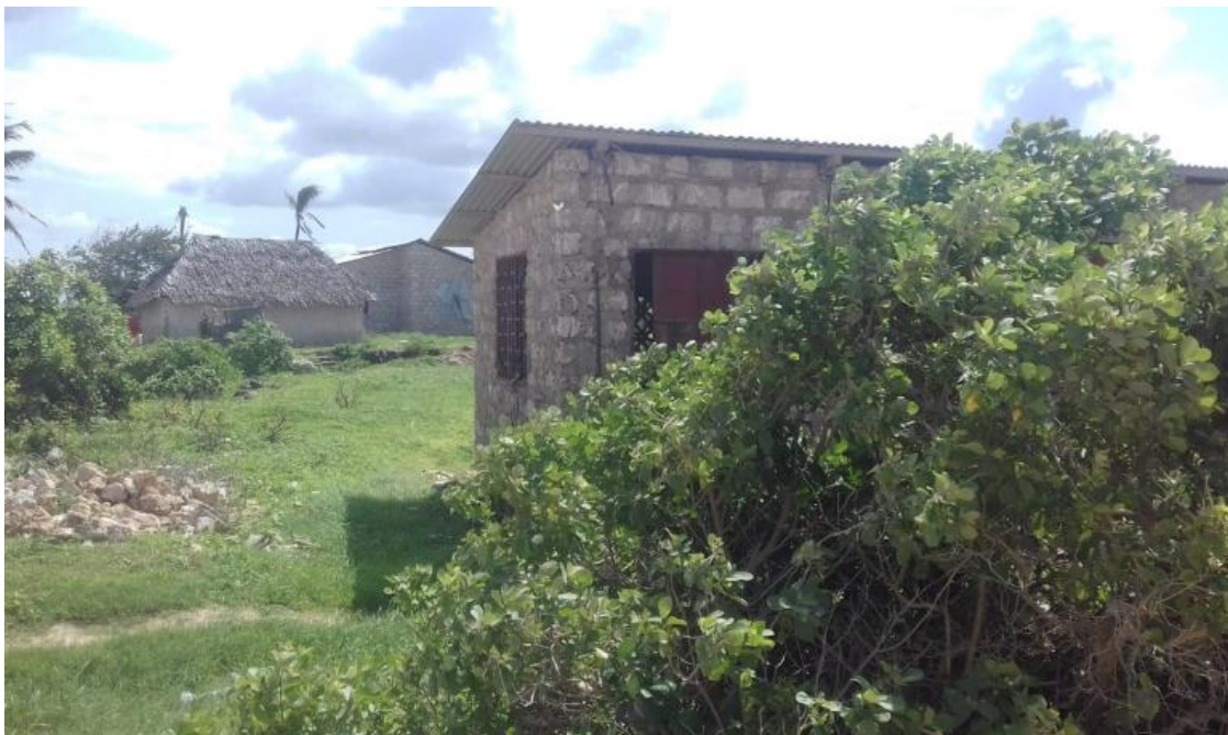
Plate 10: Residential houses built adjacent to quarry sites in Zowerani
