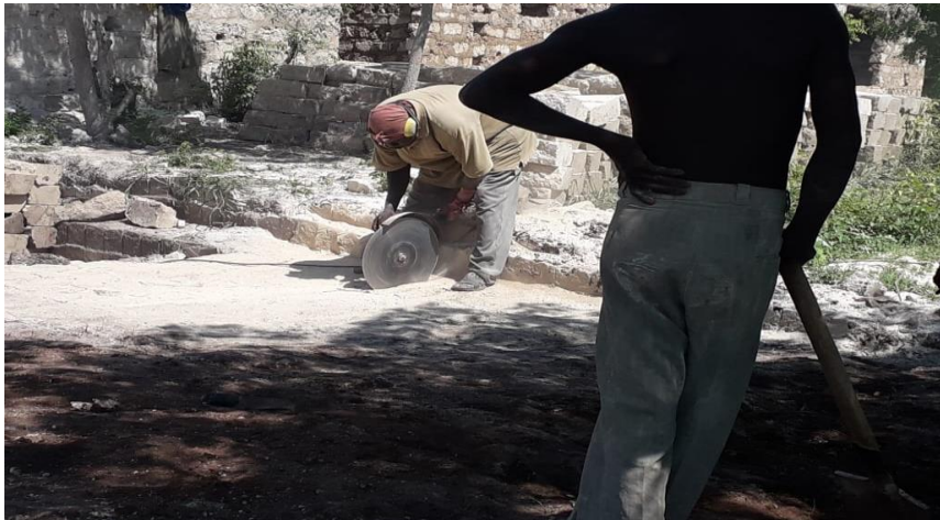
Plate 18: Stone cutting machine that produces very loud noise
