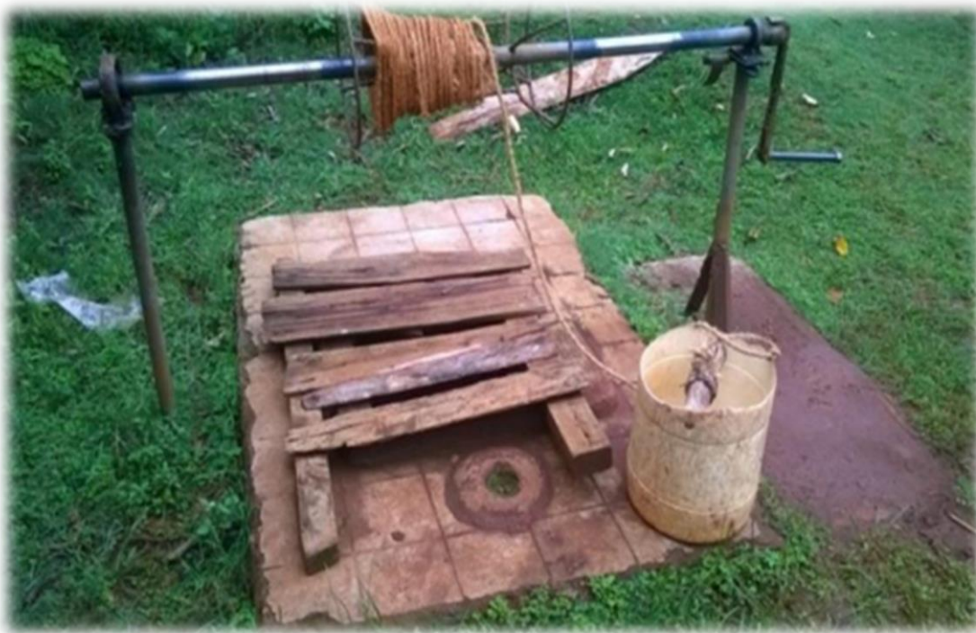
Figure 24: Shallow well in a home in Karangi for small scale irrigation
