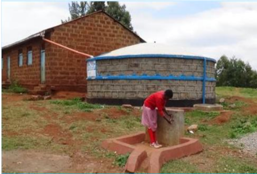
Figure 2: Rainwater storage tank
