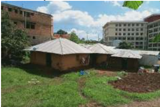
Plate 10: Dilapidated mud walled houses
