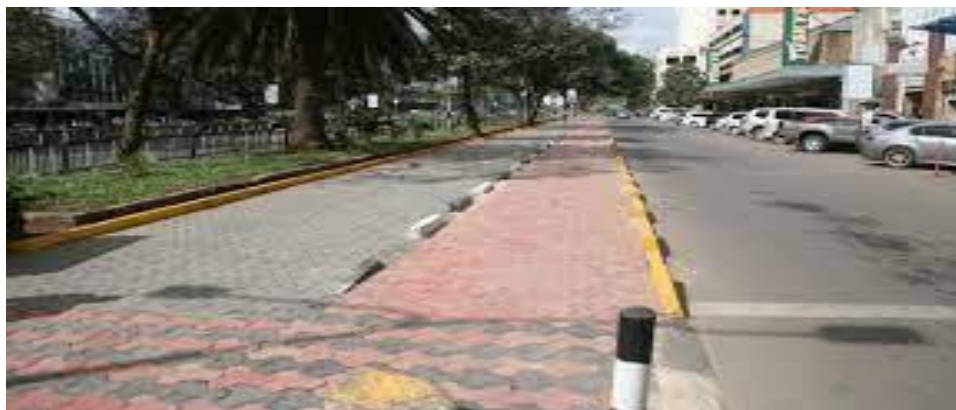
Plate 2-5: Parking spaces on the RHS of service lane converted along Kenyatta Avenue converted to NMT (Source: Nairobi Metropolitan Services)
