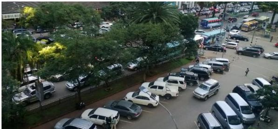
Plate 2-4: Kenyatta Avenue with Parking spaces on either side of the service lane (Source: Nairobi Metropolitan Services)
