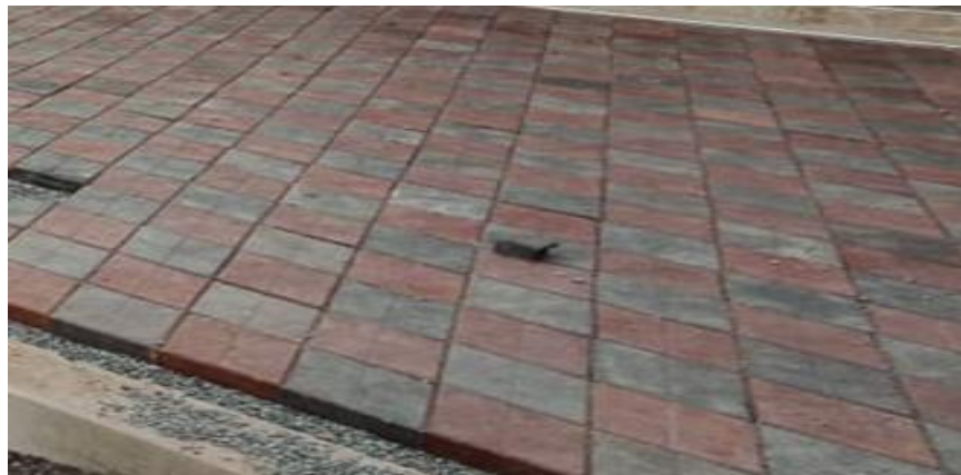
Plate 2-2: Installed Plastic Paving Blocks
