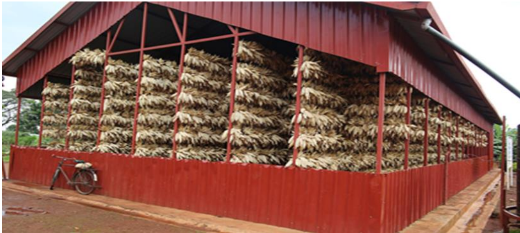
Figure 3. 2: Maize drying hanger (made of corrugated iron sheet roof and partial walls, concrete floor, and fitted with rows of metal bars from which maize on the cob is hung using the husk) Source: Gatsibo District- Agricultural division
