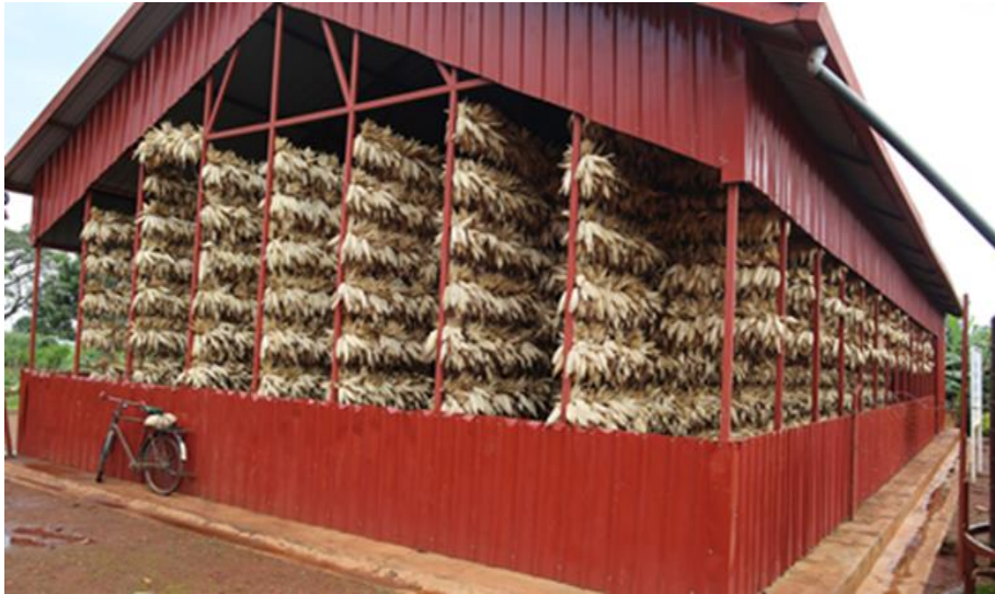
Figure 4. 3: Maize drying hanger (made of corrugated iron sheet roof and partial walls, concrete floor, and fitted with rows of metal bars from which maize on the cob is hung using the husk)
