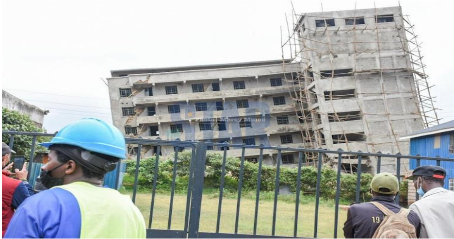
Figure 1.3: The Leaning Kinoo Building Before Demolition; Source: The Star Online, 2021
