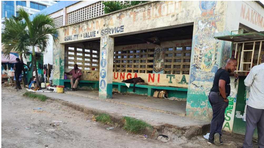
Figure 105: Bus shed along Nyerere avenue, near Naivas Likoni. Source: Author 2021
