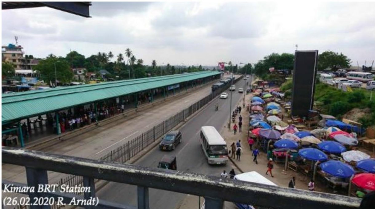
Figure 53: Aerial view of Kimara BRT Station. Source: Google images 2020
