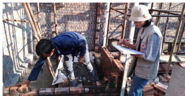
KAP Survey with a Builder Construction
