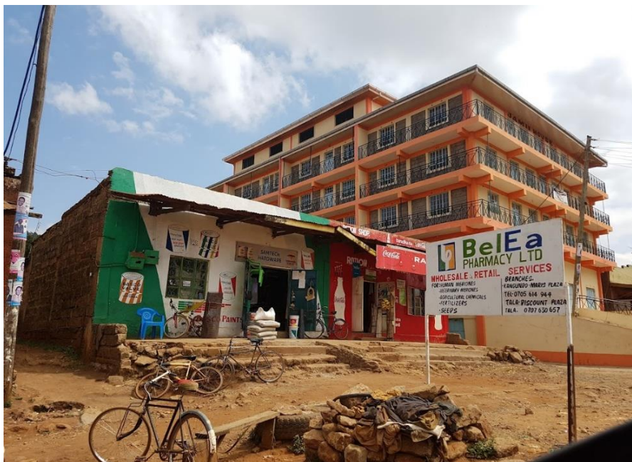
Photo 5.1: Structural Characteristics of Ruai
