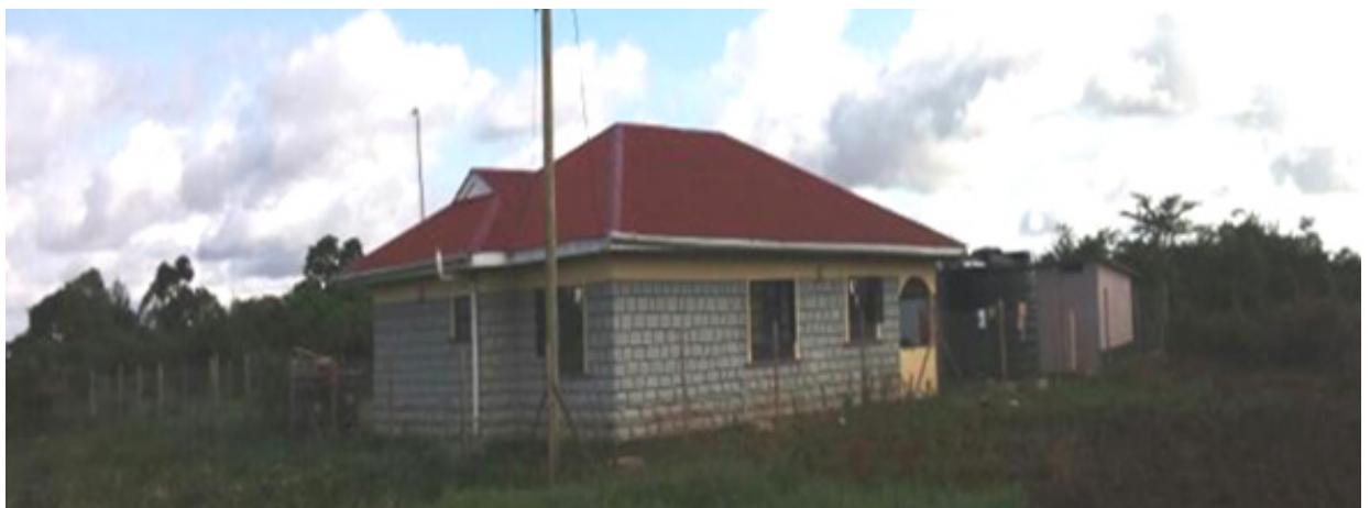
FIGURE 3 Rear view of Odhiambo residence, Sakwa Source: Qs. Belis Ochieng', 2017
