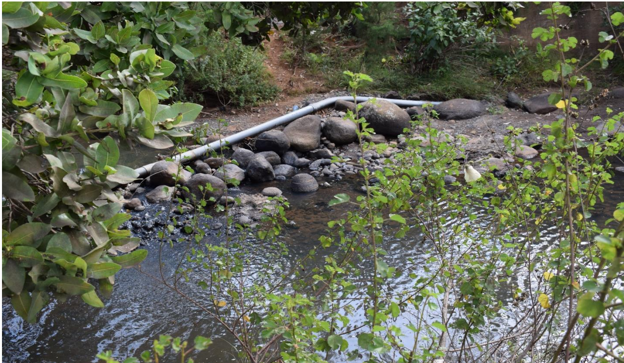
Plate 1-1: River Likii in Nanyuki town. Notice the abstraction pipe in the background.
