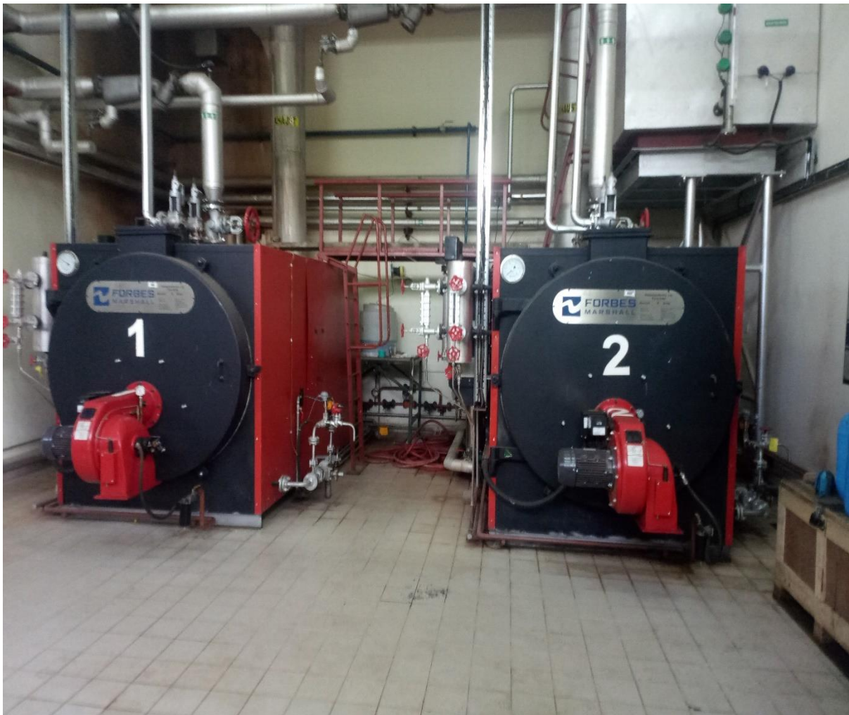
Figure 2. 3: Fire Tube Boilers [21]
