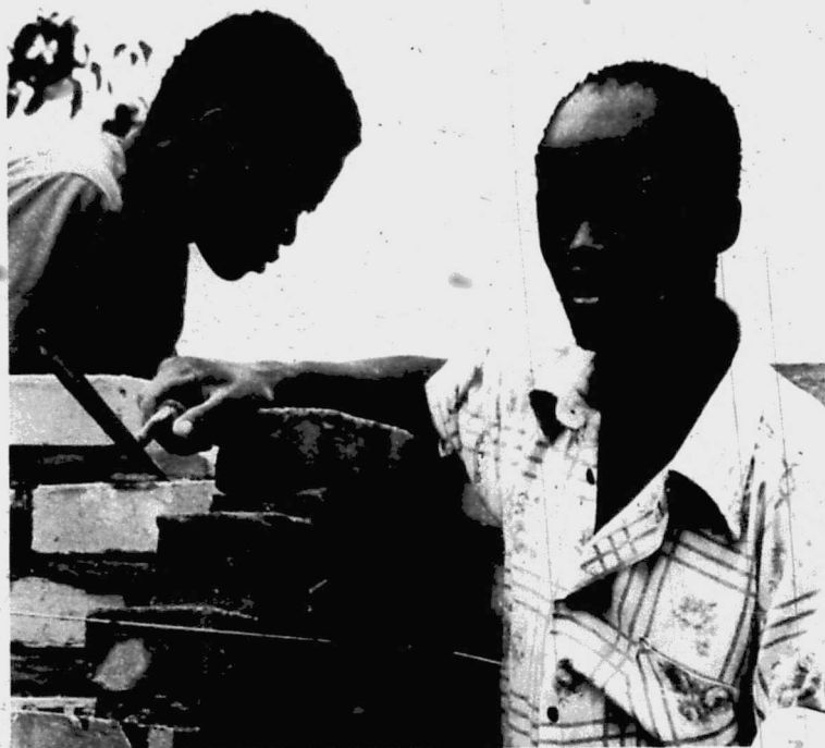
Building trainees construct new staff housing, financed by the World Bank
