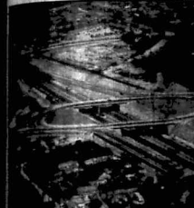
At the worst of times on Britain's Great North Road — the City of Doncaster — ended in 1957 with the opening of a £2,000,000 bypass. This aerial picture shows a section of the new bypass, which have been built up to motorway standards. Thirty bridges had to be built by the British by sea, which will eventually link up with the London-Yorkshire Motorway.
