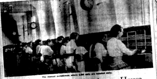
The manual switchboard where 4,500 calls are handled daily.
