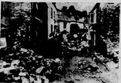
This was how the picture-postcard village of Preed, Somalia, looked after raging Red waters had reared havoc through the village at a level of eight feet and several houses collapsed into the river. The village has been named a "disaster area." At least seven persons died in the flooding which swept through the West of England. The flooding followed 24 hours of torrential rain.
