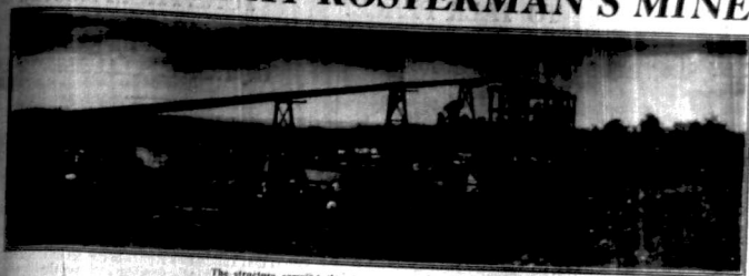
The structure carrying the conveyor belt to the stamping mill.
