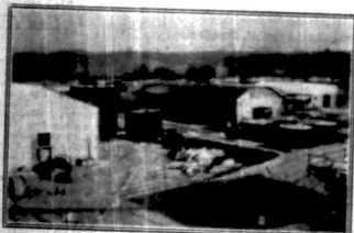
Looking down on the Power house, Oil storage tanks, Workshops, etc.
