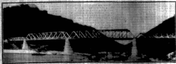
The great Ruaha Bridge of 4 spans with a total length of 405 feet on the Kilosa-Ikaka Road. Photo: C. V. Stevenson.
