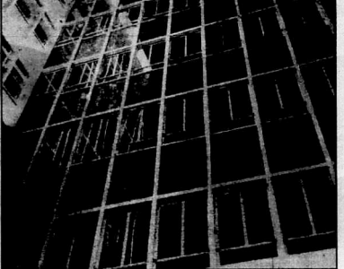
Green glazed-tile panels between white concrete ribs which form the new building facade make an attractive pattern against Nairobi's blue sky.
