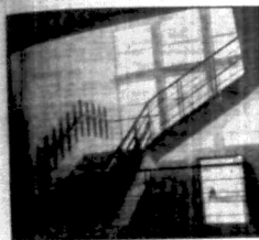
Several heavy double-glazed aluminium doors are set in an anti-bombing design. Shaded by slats, at the main entrance, is the first floor of slats as seen from the tower. The building is built in brick with slats and pillars finished in aluminium. A section of the anti-bombing operations in the building is shown in the tower. All windows are made of double glazing to make full use of 1,000 square feet of wall space for hanging maps.
