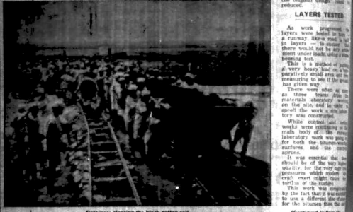
Contractors clearing the beach section soil.
