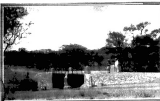
Another view of the Mbeya bridge
