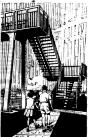
Footbridge fabricated in R.H.S. by Tubewrights Ltd. and supplied to the Government of Northern Ireland. This structure can be readily dismantled and re-erected on an alternative site. Its length can be extended by the introduction of additional spans. Similar footbridges are under construction for erection in Holland.
