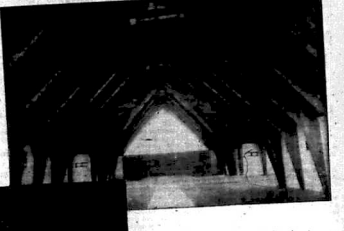
The Roman Catholic Church at Thomson's Falls was constructed almost entirely of timber supplied by the Timms-Jarvis Group. This building is an example of the many ways timber can be adapted to suit the most modern architectural designs.
