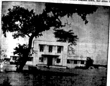
An old tree forms a pleasant frame for the modern council offices at Kitale.
