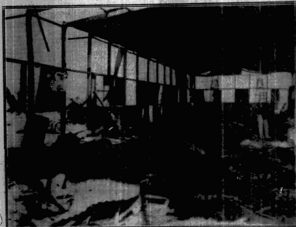
One of the gutted workshops on the aerodrome of El Adem.
