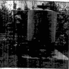
This sand filter, with a small electric pump to push the water through it, ensures that the water is crystal clear. A diagram showing the working of the filter in Page 18.
