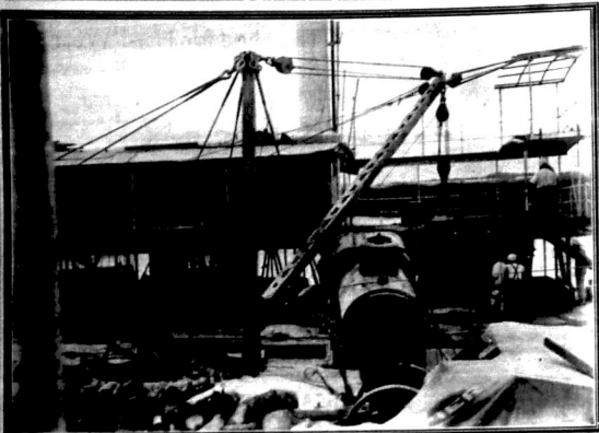
ENGINEERING FEAT AT BUTIARA. S.W. Logard's engine, being repaired under the management of Commander Lockhart and Mr. ...
