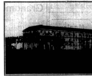
The Government Central Offices.
