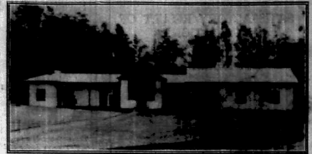
The Health of the African: Maternity block at Kisumu Native Hospital.
