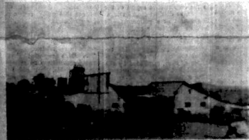
Kenya Gold Mining Syndicate's new Crusher and Power Station.
