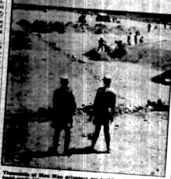
Thousands of African prisoners are building the world's first hand-made international airport at Embakasi. It is equal in size to the airport at Addis Ababa. One end of the runway (see inset) is used as an experimental area for laying and testing the final surface.
