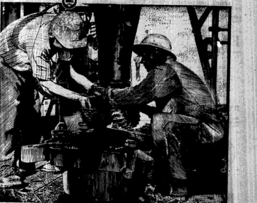
Getting ready to start drilling. The bit is cleaned and then attached to the drill pipe and screwed fast.
