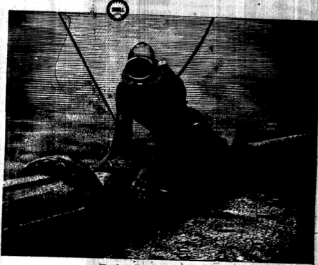
The flexible hose connections of a 18-inch diameter pipeline being inspected by a diver. This pipeline speeds the discharging and turn-round of tankers
