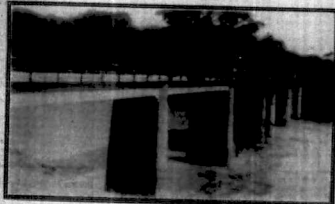
A view of the new concrete bridge over the Great Ruaha River on the Kilosa-frings road of Tanganyika. The Bridge has a length of 344 feet and carries a 10-foot roadway with a 2' 6" footpath on each side. C. V. Stevenson.
